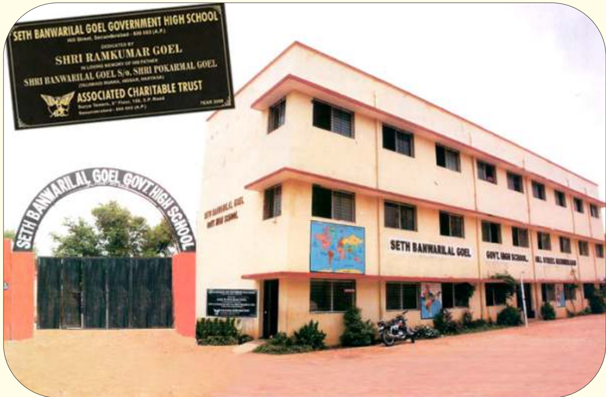
Construction of SETH BANWARILAL GOEL GOVT. HIGH SCHOOL at Hill Street, Secunderabad (Telangana), under public-private partnership with Sarva Siksha Abhiyaan.
