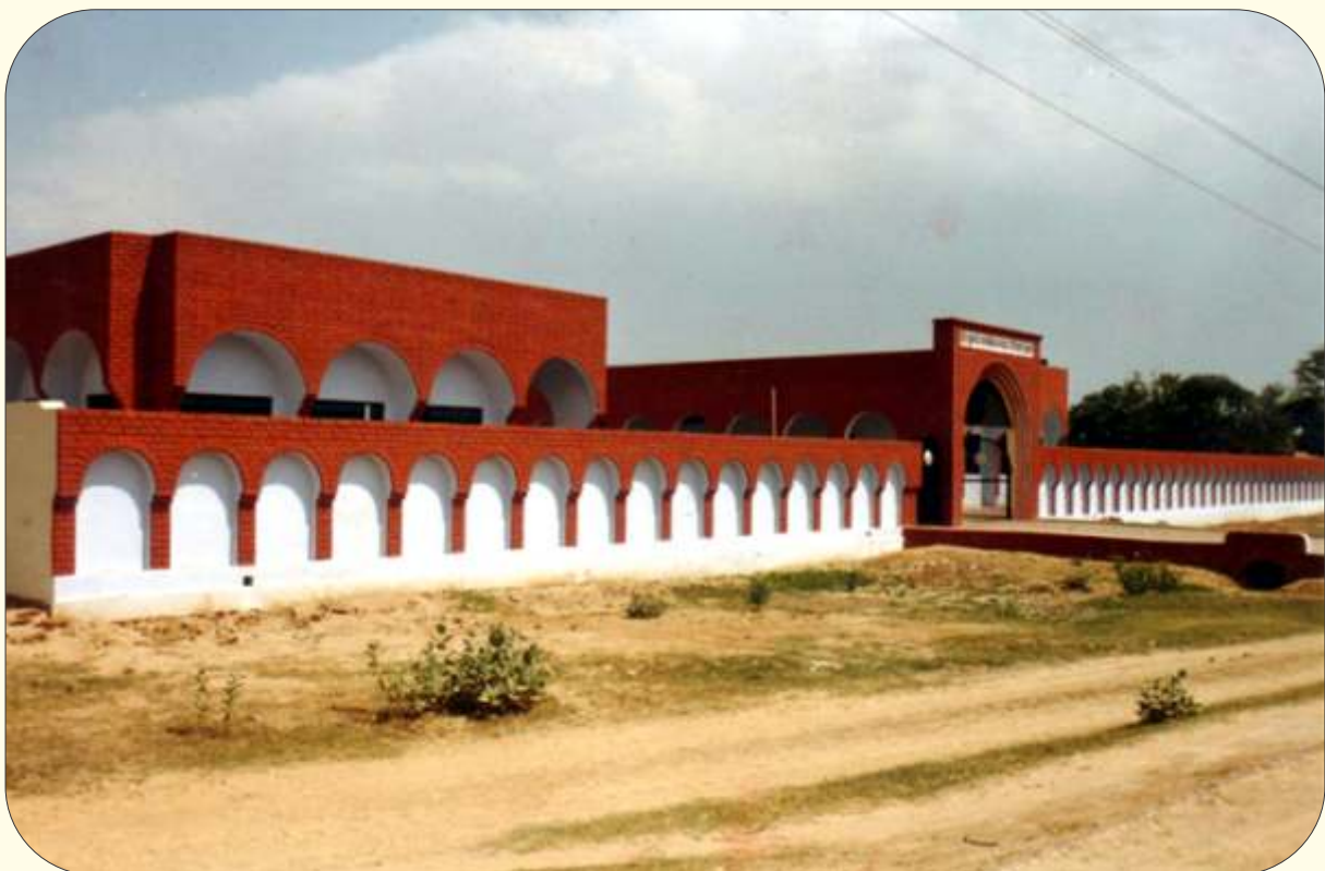
SETH MULCHAND RAMJILAL RAJKIYA MADHYAMIK VIDYALAY, Bugana (Haryana) - Constructed and donated by Associated Charitable Trust.
