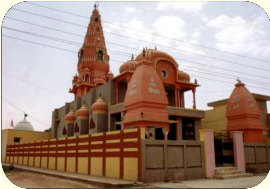
Construction of SHREE RAM MANDIR at Talwandi Rukka, Hissar (Haryana)
