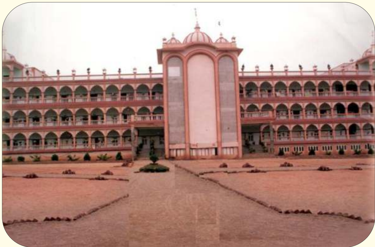
Construction of a block in the hostel of SRI SWAMI NARAYAN GURUKUL in Moinabad, Hyderabad (Telangana).
