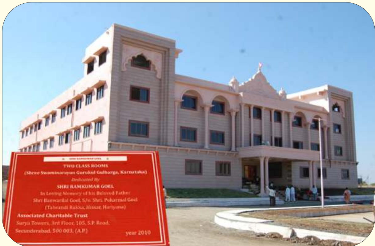
Construction of Two Class Rooms at SHREE SWAMINARAYAN GURUKUL, Gulbarga (Karnataka).
